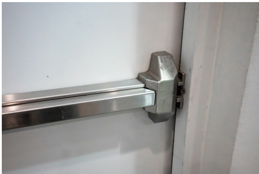
Figure 7-4. Example image of door with push bar—interior view (not image of door at Robb Elementary)
