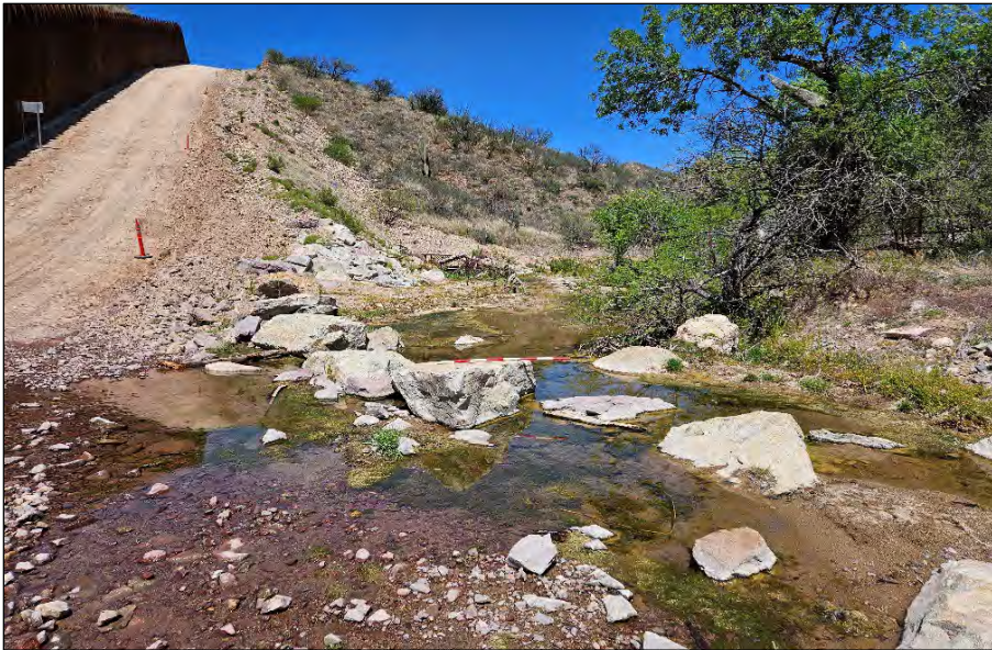
Drainage 47, Photo 3. Looking upstream, facing northwest.
