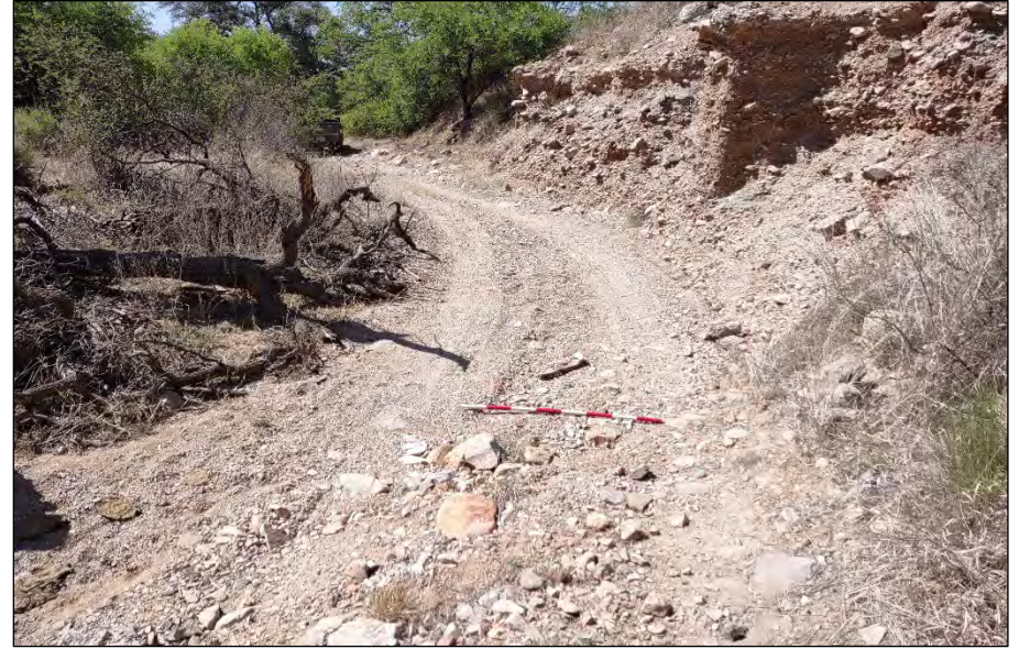
Drainage 29, Photo 14. Looking downstream, facing south-southeast.
