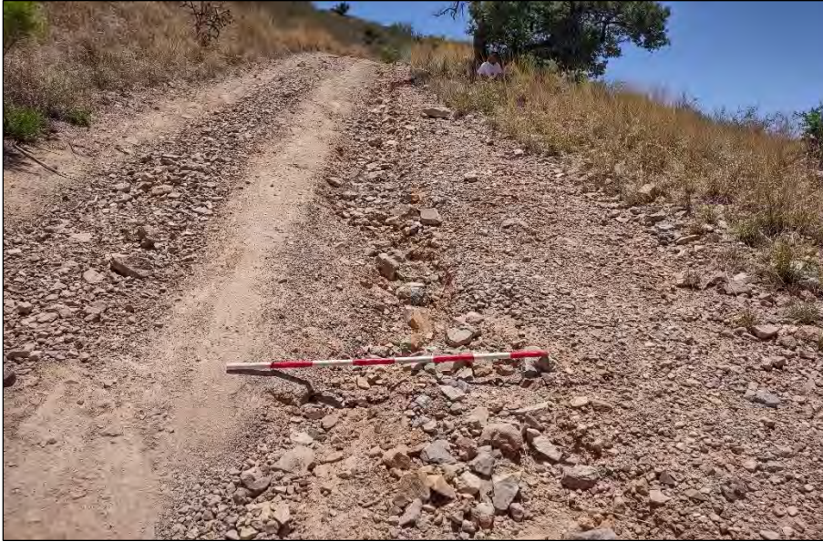
Drainage 27, Photo 1. Looking upstream, facing south.
