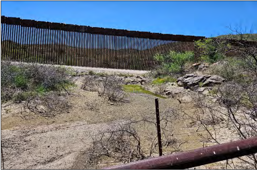
Drainage 52, Photo 1. Looking downstream, facing southwest.
