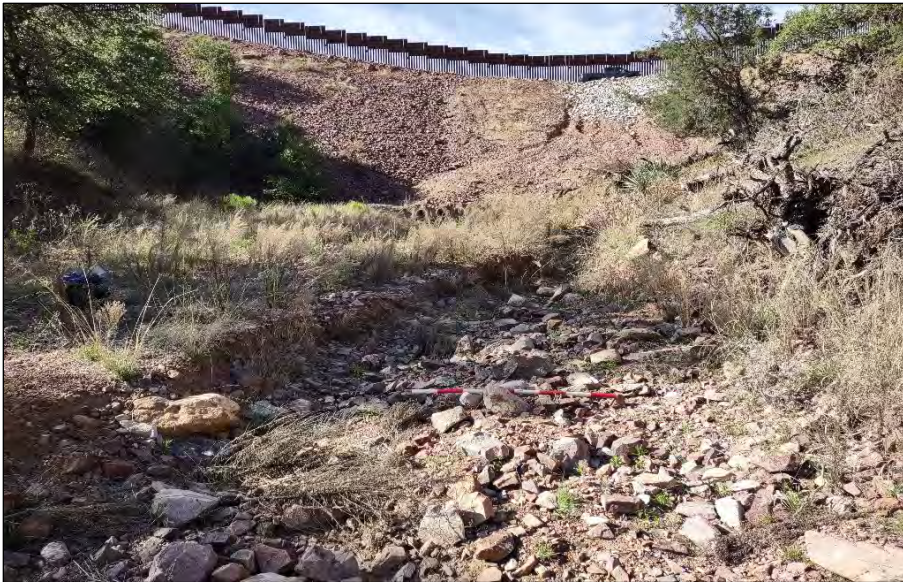
Drainage 55, Photo 1. Looking upstream, facing south.
