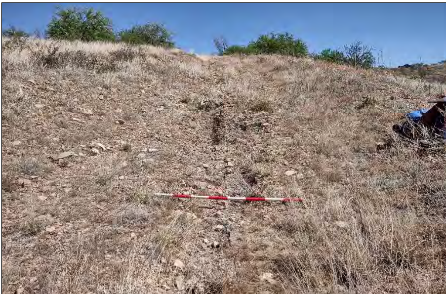
Drainage 7, Photo 1. Looking upstream, facing northeast.
