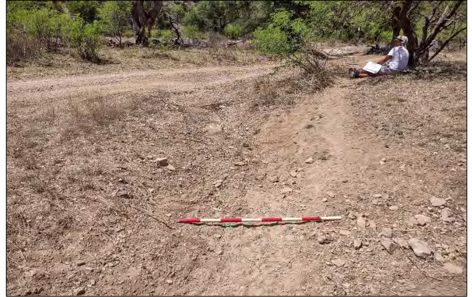
Drainage 24, Photo 2. Looking downstream, facing southwest.
