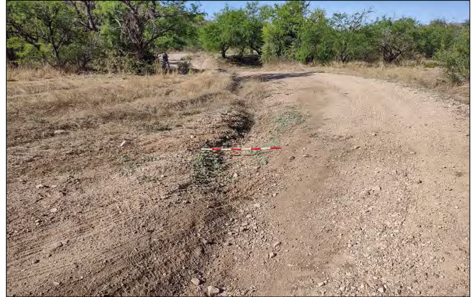
Drainage 17, Photo 2. Looking downstream, facing south-southwest.
