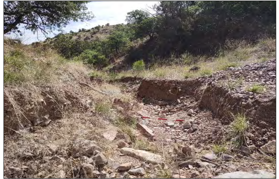
Drainage 53, Photo 2. Looking downstream, facing northeast.
