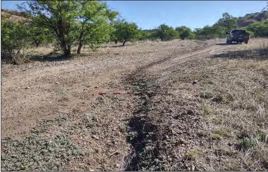
Drainage 17, Photo 1. Looking upstream, facing northeast.
