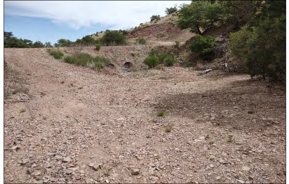
Drainage 53, Photo 6. Looking downstream, facing northeast.
