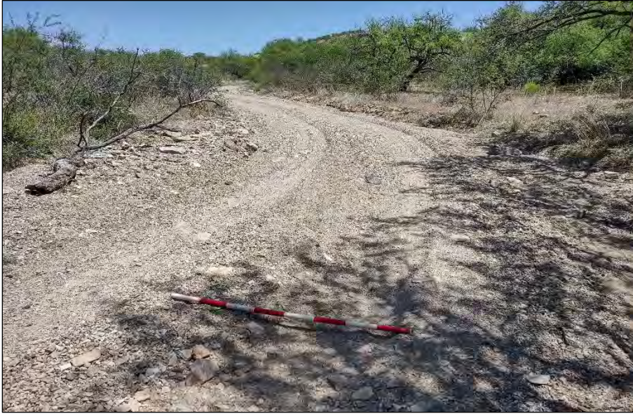
Drainage 29, Photo 21. Looking upstream, facing north-northeast.
