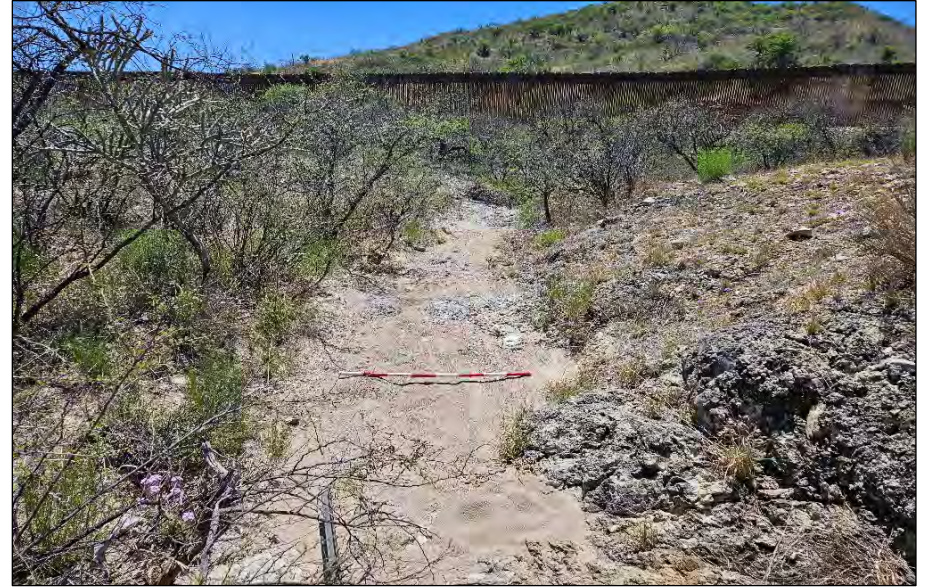
Drainage 48, Photo 2. Looking downstream, facing southwest.
