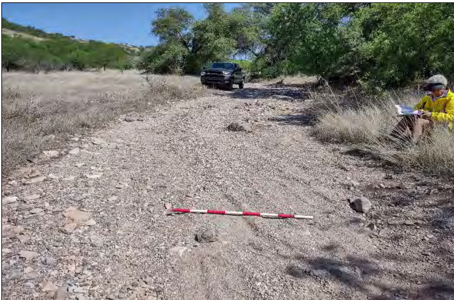
Drainage 29, Photo 15. Looking upstream, facing north.
