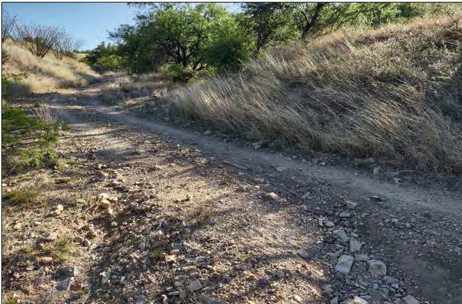
Drainage 28, Photo 1. Looking upstream (no upstream), facing east-northeast.
