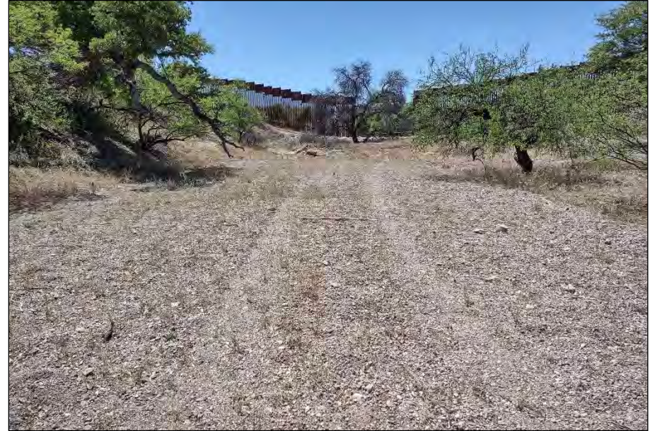
Drainage 3, Photo 2. Looking downstream, facing south-southeast.
