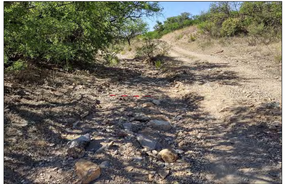
Drainage 29, Photo 8. Looking downstream, facing south-southeast.
