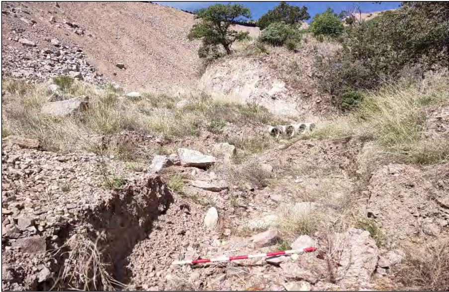
Drainage 53, Photo 1. Looking upstream, facing southwest.
