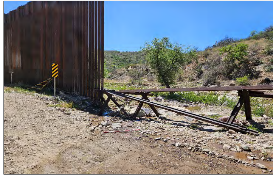
Drainage 47, Photo 4. Looking downstream, facing southeast.
