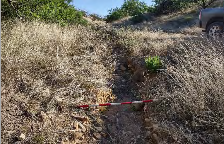
Drainage 28, Photo 3. Looking upstream, facing north-northeast.
