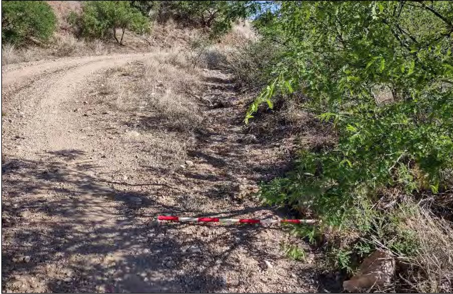
Drainage 29, Photo 1. Looking upstream, facing northeast.
