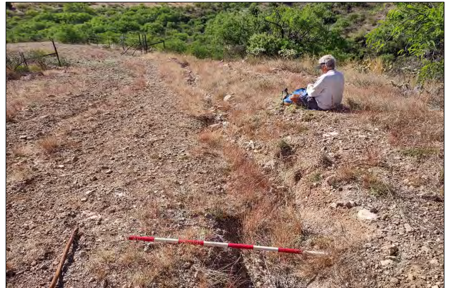
Drainage 9, Photo 2. Looking downstream, facing southeast.
