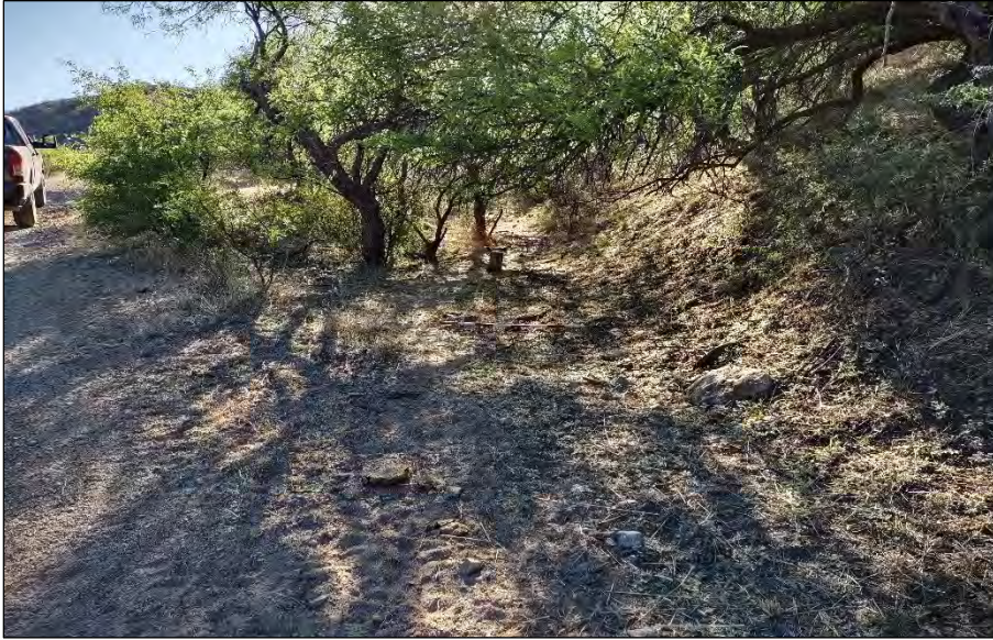
Drainage 14, Photo 1. Looking upstream, facing east.
