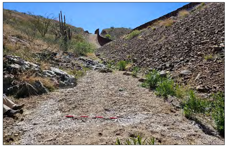
Drainage 42, Photo 6. Looking downstream, facing east-southeast.
