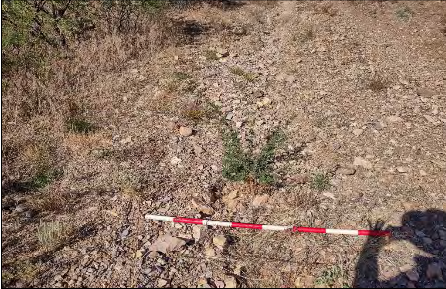
Drainage 8, Photo 1. Looking upstream, facing southwest.
