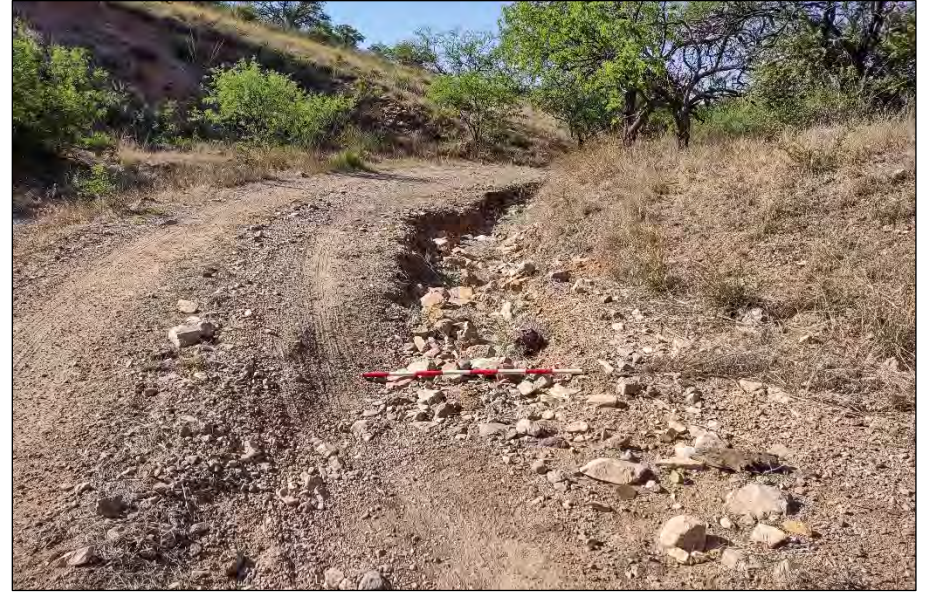
Drainage 29, Photo 2. Looking downstream, facing south-southwest.
