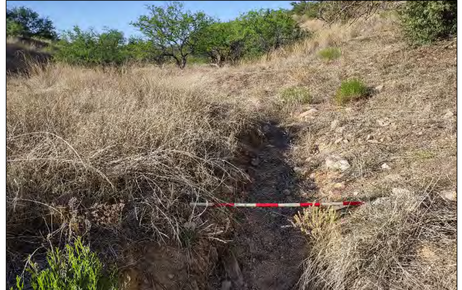
Drainage 28, Photo 4. Looking downstream, facing south.
