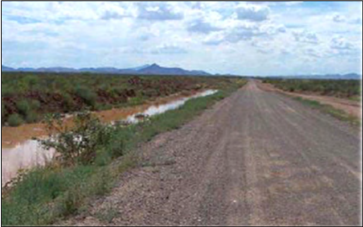
Figure A-3. FC-2 All-Weather Road (Photograph)
