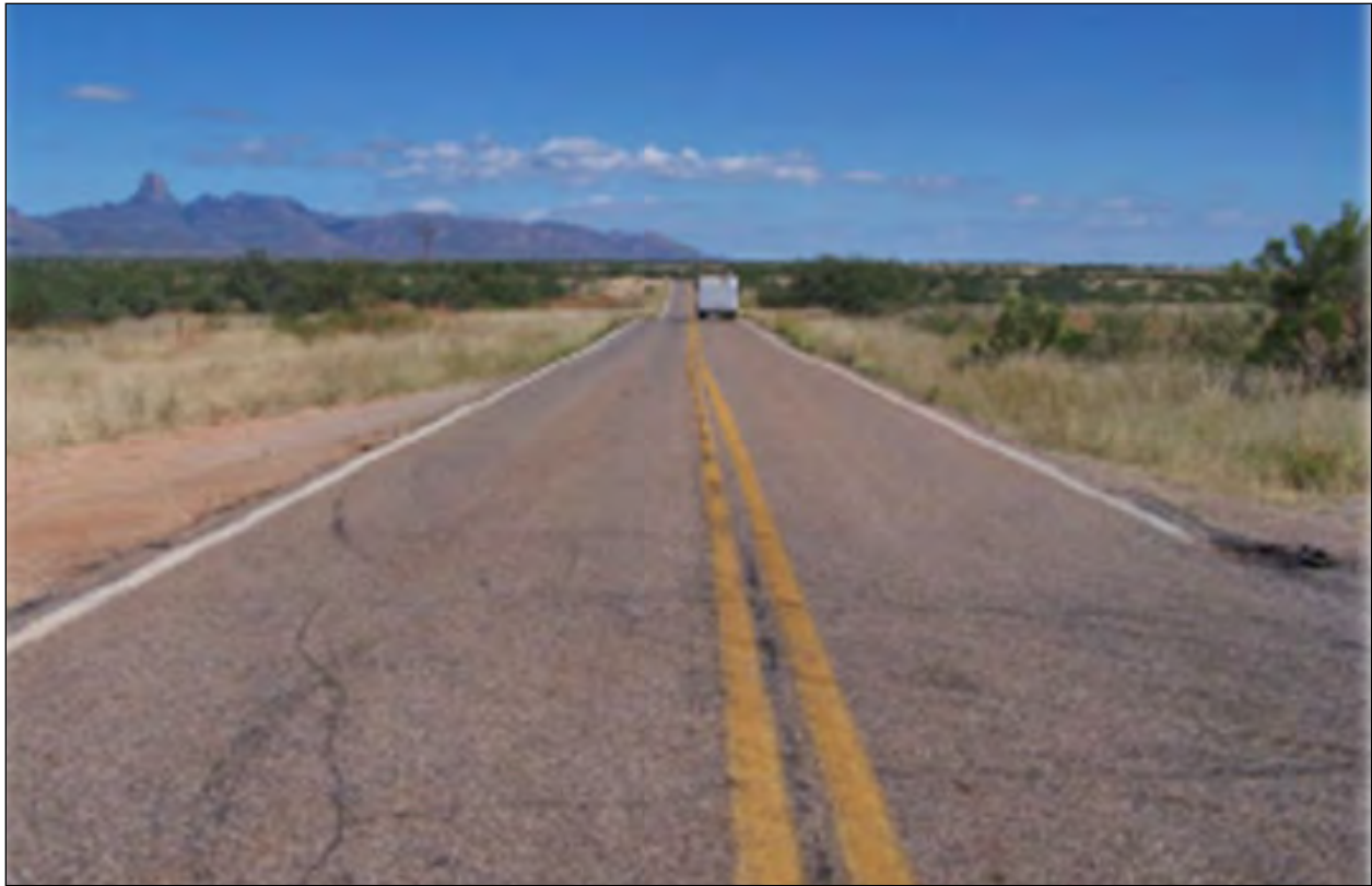
Figure A-1. FC-1 Paved Road (Photograph)
