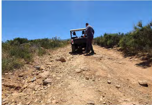
Water Cutout (WC6)
