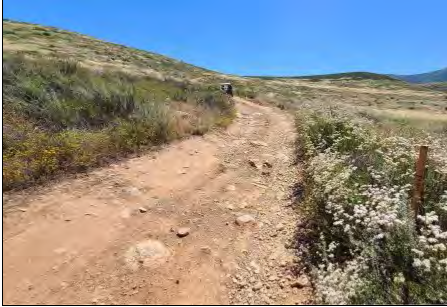
Photograph 2-1. Example Water Bar Location
