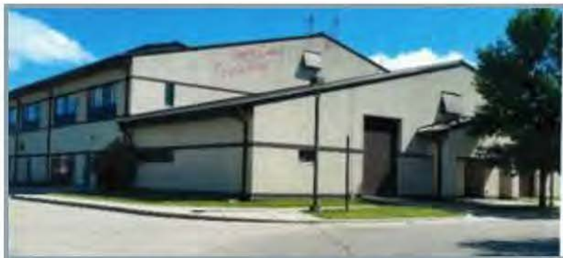
Relocation of UAV' Operations , Classroom and Flight Instruction, Parts Warehousing and Administration from (b) (7)(E) (b) (7)(E)
