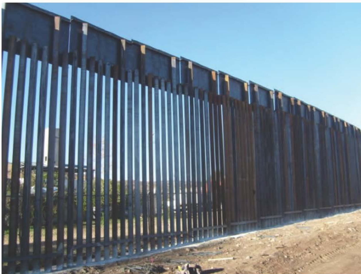
Pedestrian Fence – (b) (7)(E) Tucson Sector
