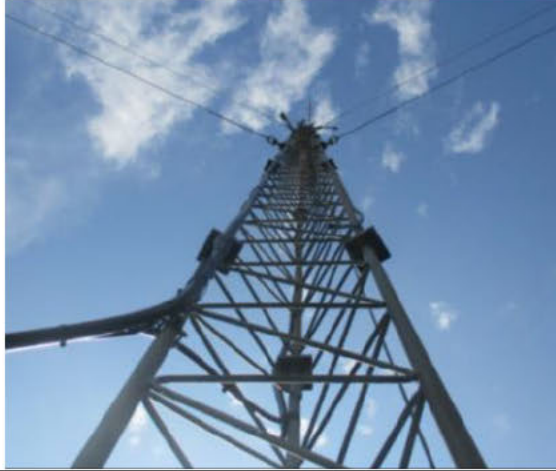
(b) (7)(E), (b) (5) . Install lightning protection. (b) (7)(E)
