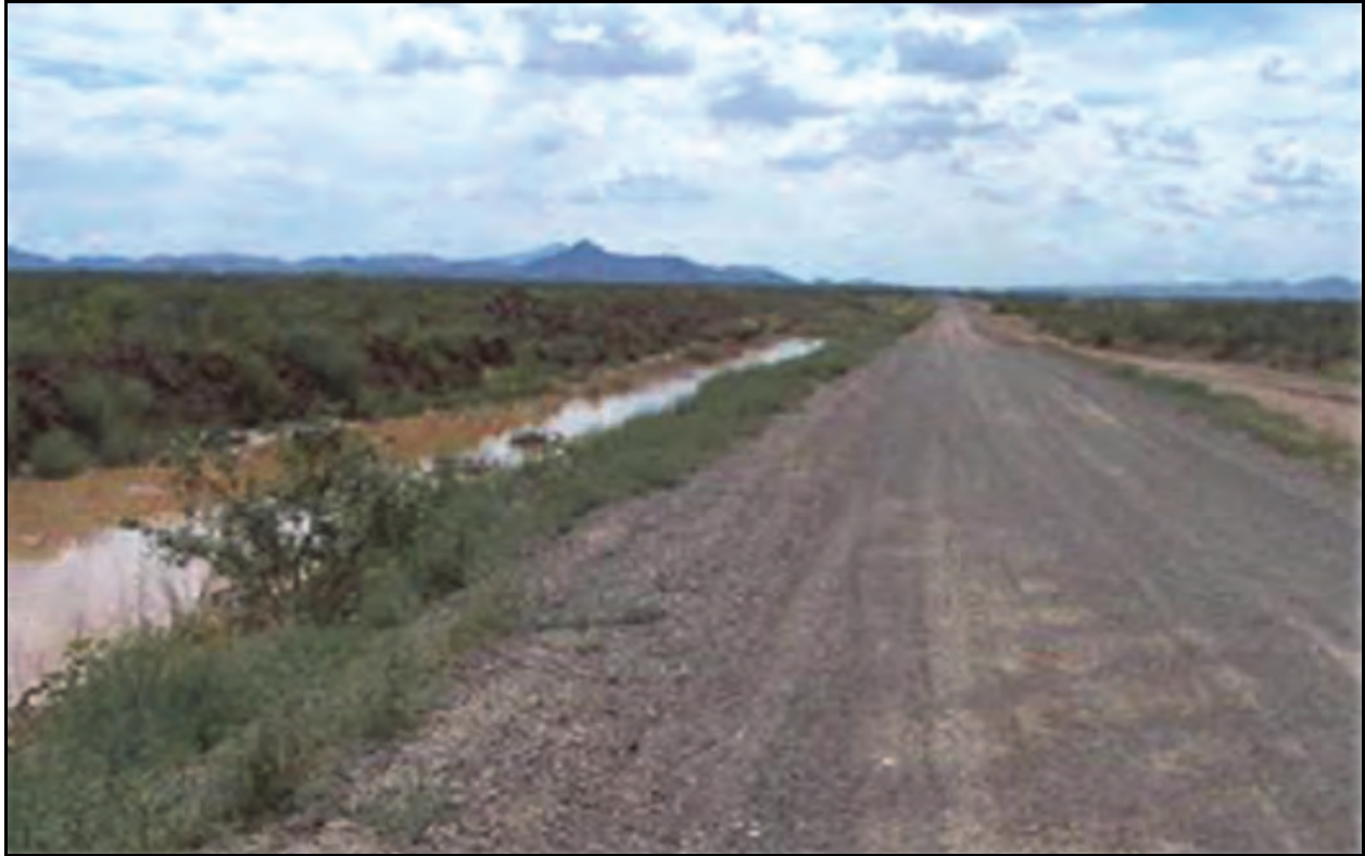
Figure C-3. FC-2 All-Weather Road (Photograph)
