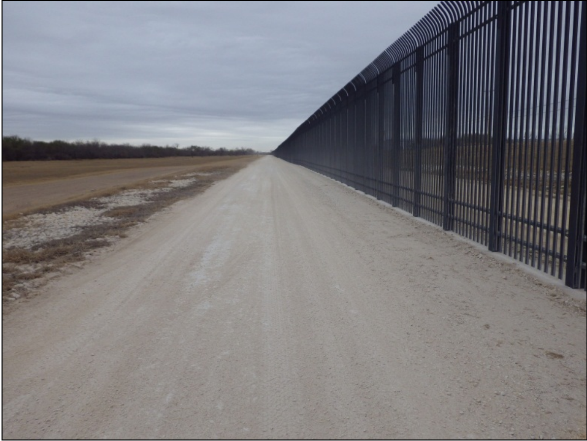
Figure C-3. FC-2 All-Weather Road (Photograph)
