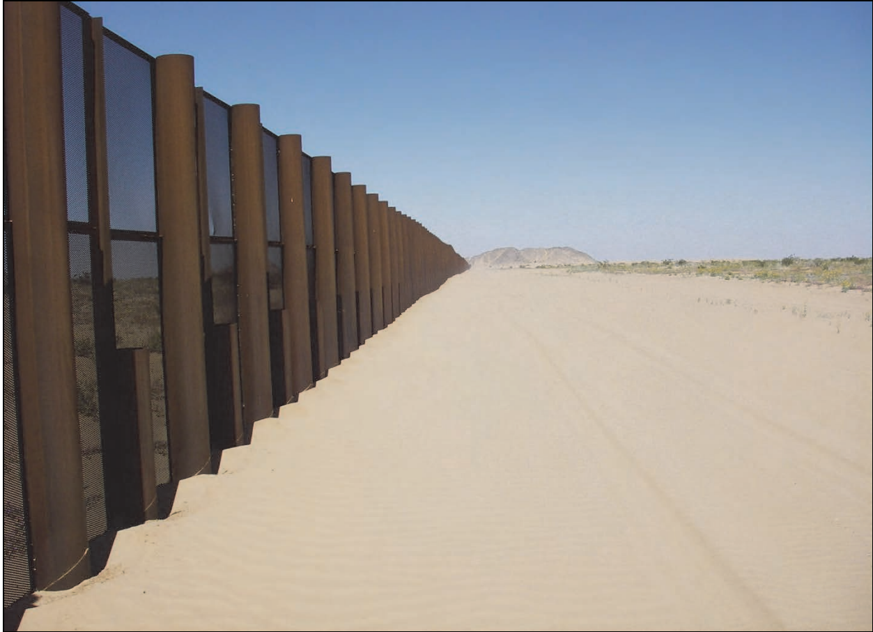
Figure C-9. FC-5 Sand Road (Photograph)
