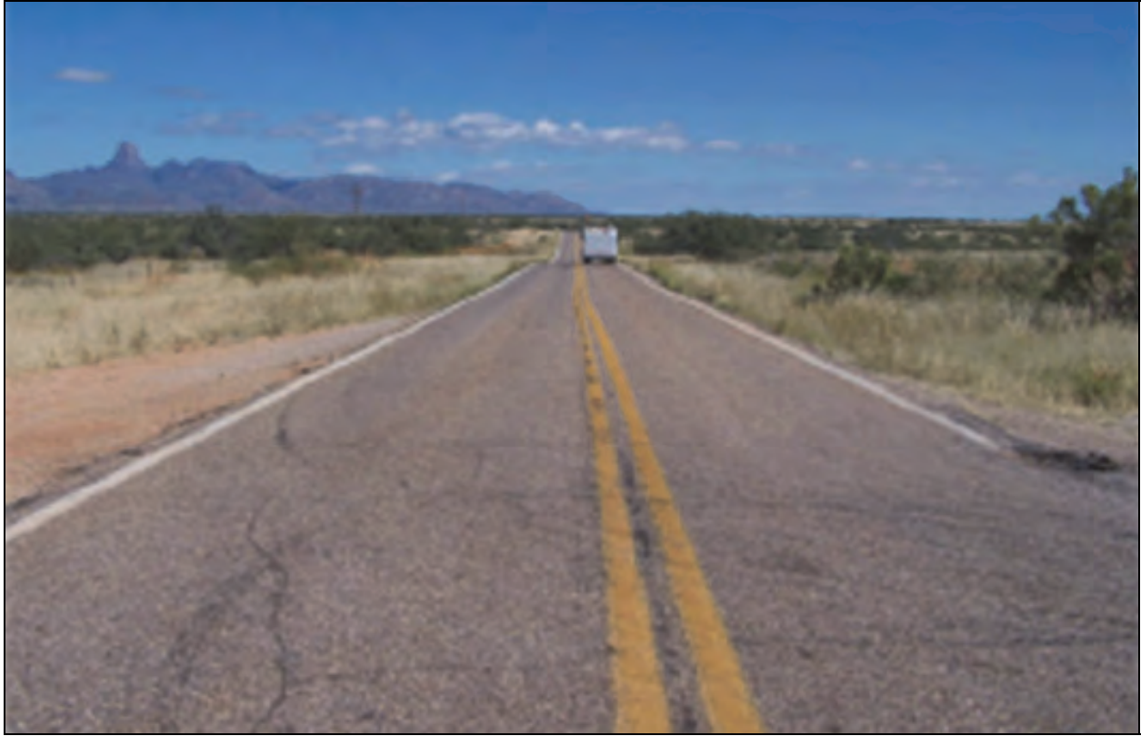
Figure C-1. FC-1 Paved Road (Photograph)
