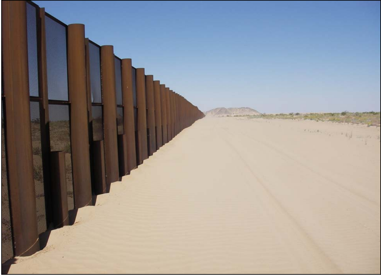
Figure C-9. FC-5 Sand Road (Photograph)
