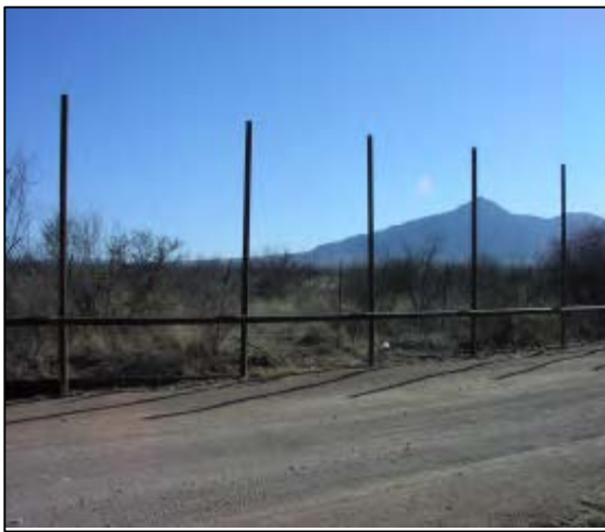
Permanent Vehicle Barrier with 10-foot Fence Extensions
