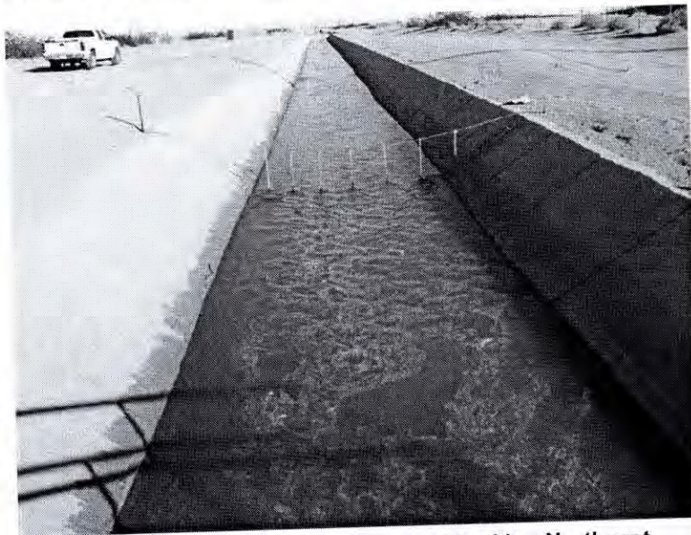
Photograph 1: 242 Well Field Canal looking Northeast
