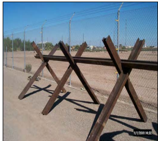
Temporary Barrier Constructed from Railroad Rails
