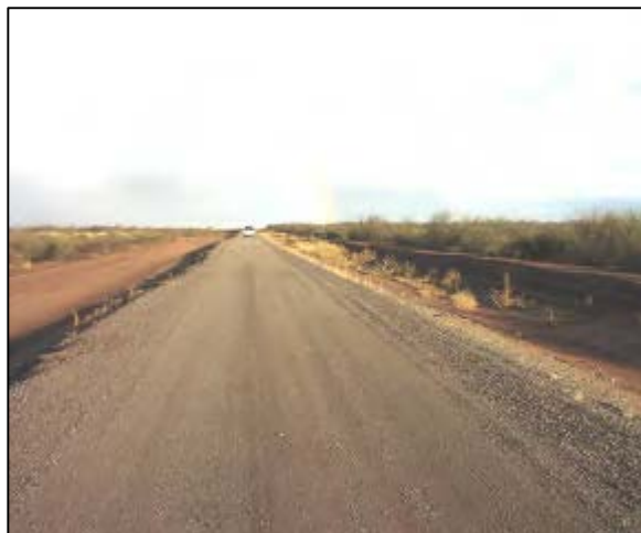
Photograph 1-17. Border Road with Improvements
