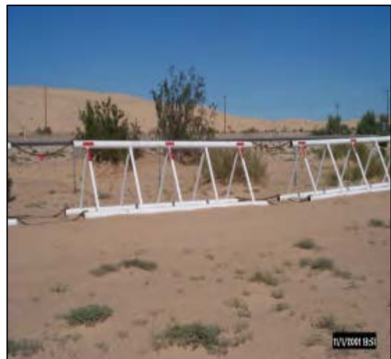
Temporary Barrier Constructed from Pipe
