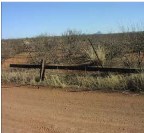
Permanent Low Vehicle Barrier
