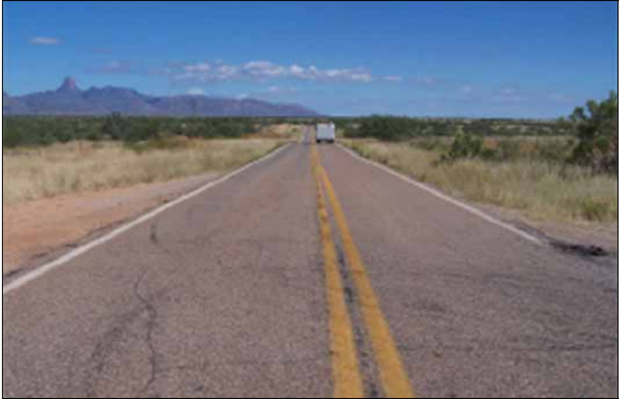
Figure C-1. FC-1 Paved Road (Photograph)
