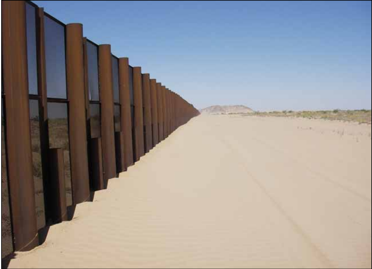
Figure C-9. FC-5 Sand Road (Photograph)
