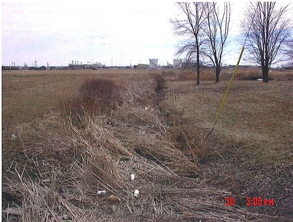
Reach of drainage ditch – looking downstream from Lockport Road
