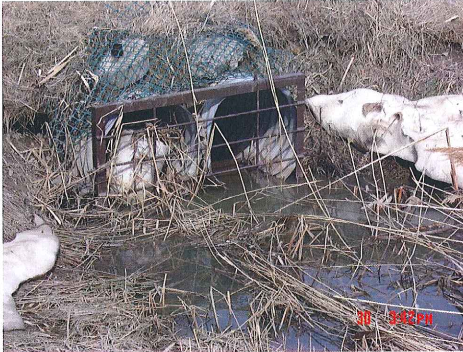
Downstream side of culvert
