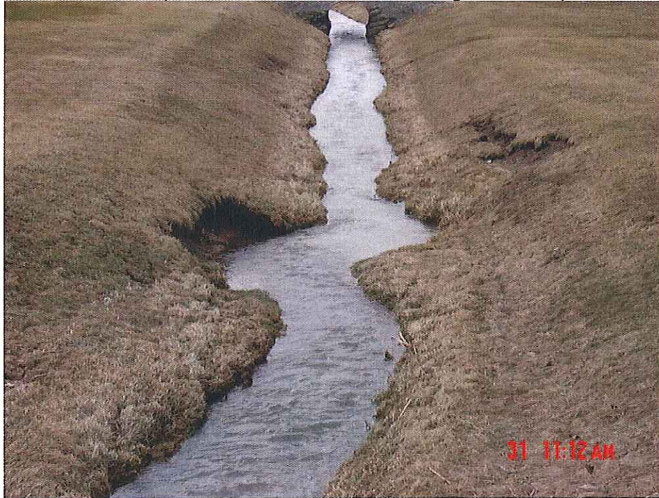
Channel section between Bridges #4 & #5 – location of cross section #9
