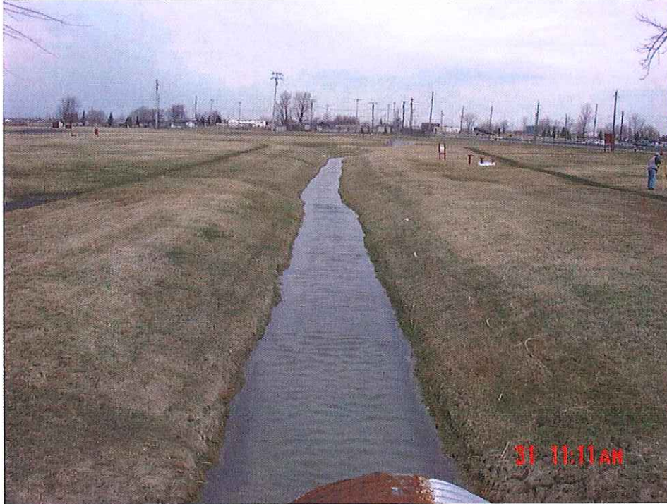
Looking upstream through cross section #7 from bridge #3
