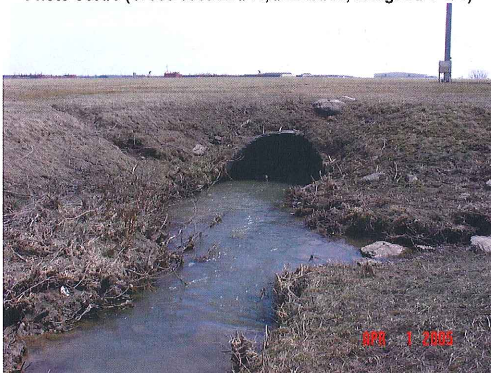
Upstream face of Bridge #8
