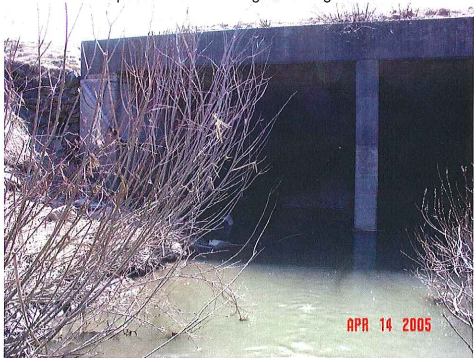
Upstream face of bridge #10 – left half
