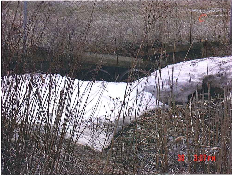
Upstream side of bridge #1
