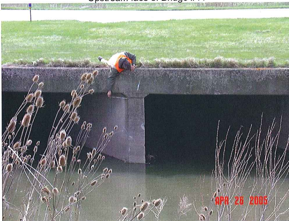
Closer look at upstream face of bridge #11
