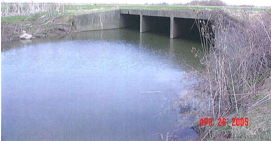
Downstream face of bridge #18
