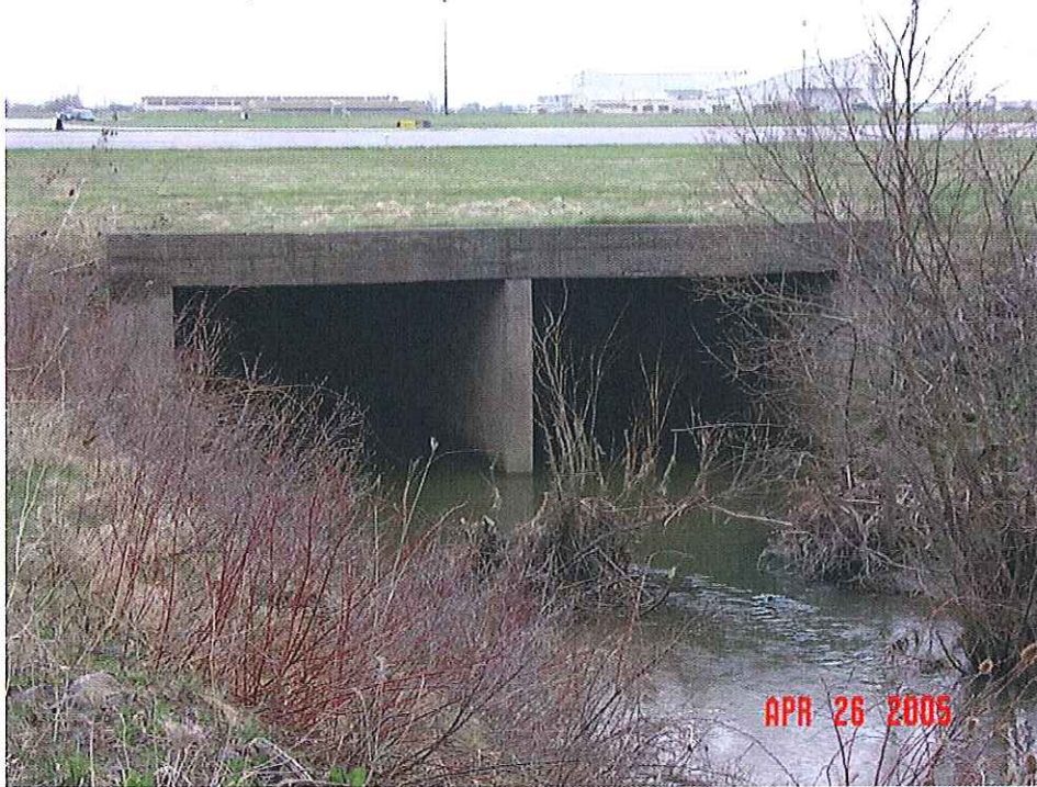
Downstream face of bridge #10
