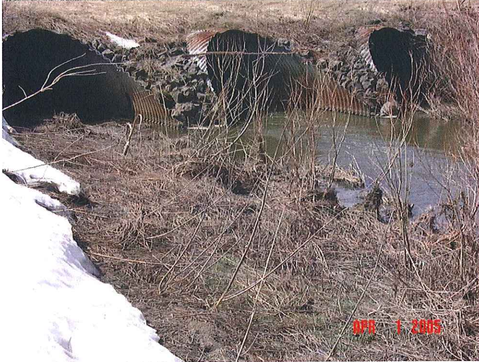
Upstream face of bridge # 9
