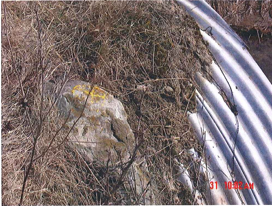
Location of temporary bench mark, downstream side of culvert
