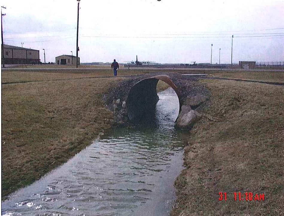
Upstream face of bridge #3
