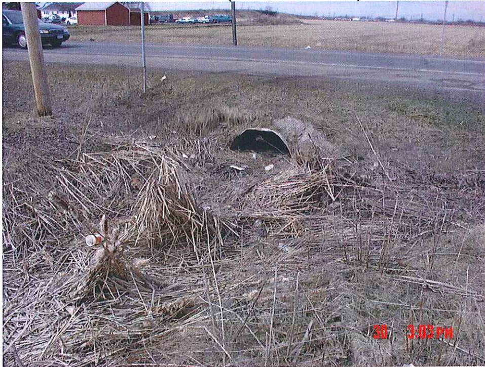
Culvert under Lockport Road (downstream side)
