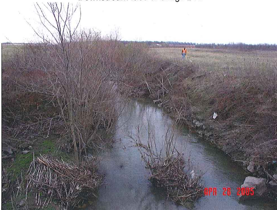
Looking downstream from bridge #10
