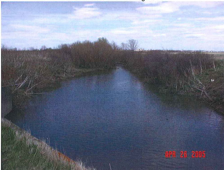
Looking upstream from bridge #11
