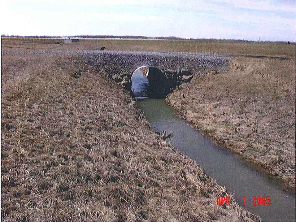
Upstream face of bridge #7
