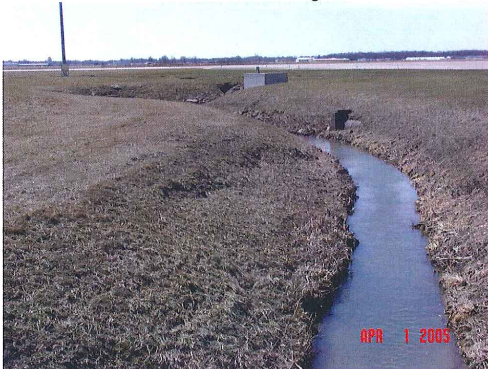
Looking downstream from bridge #7 cross section #13 is located in this reach
