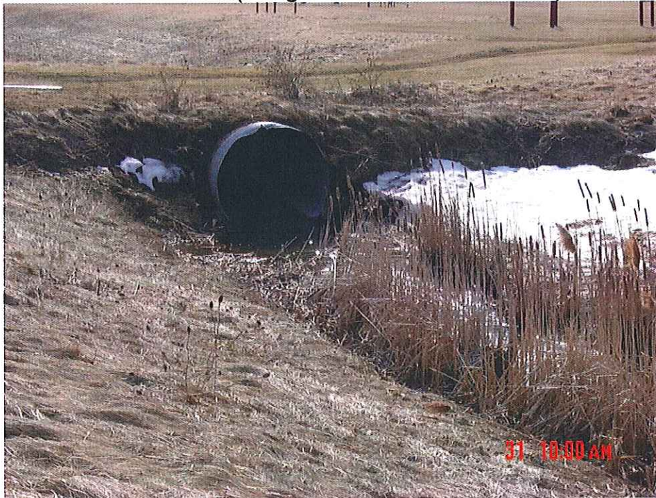
Upstream side of culvert identified as bridge #2
