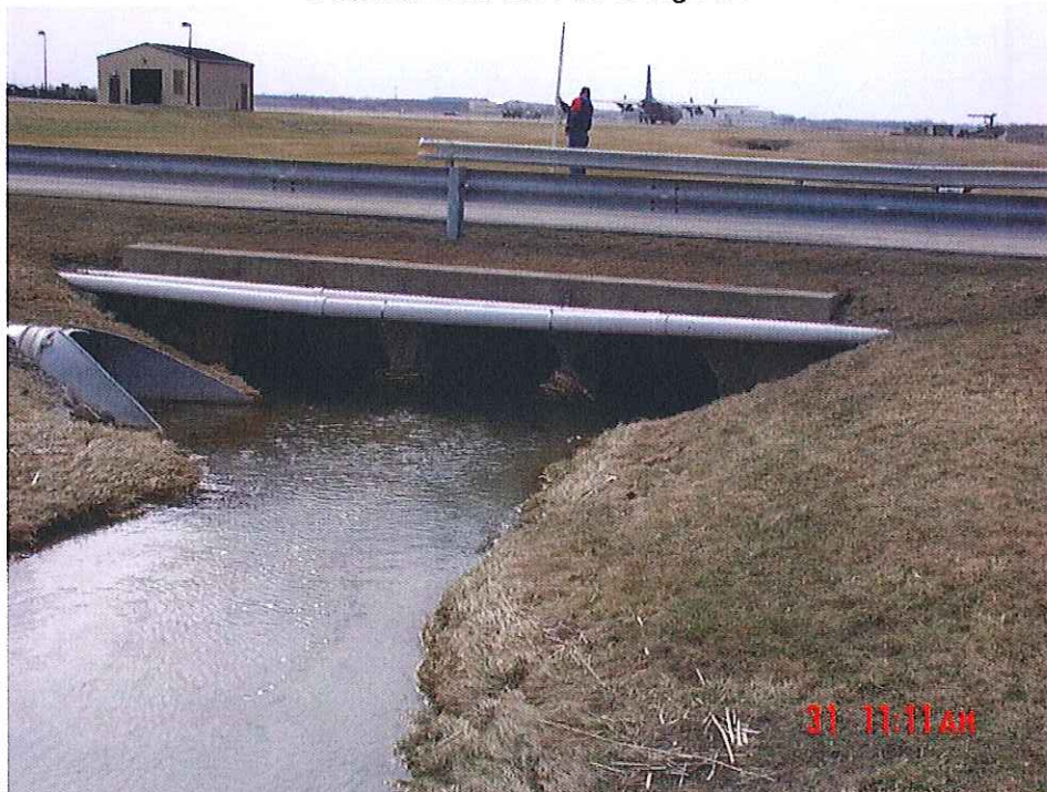
Upstream face of bridge #4
