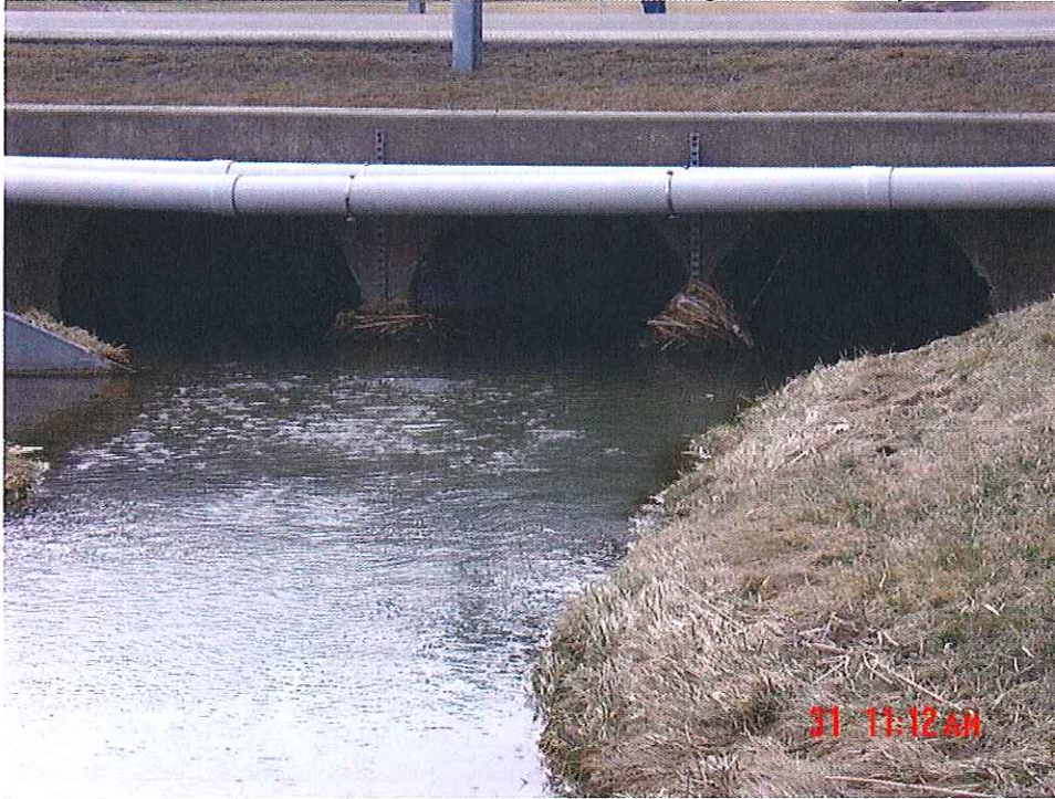
Closer view of upstream face of bridge #4
