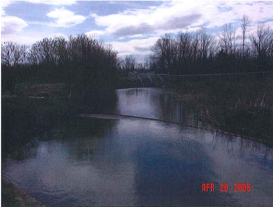
Looking downstream from bridge #11
