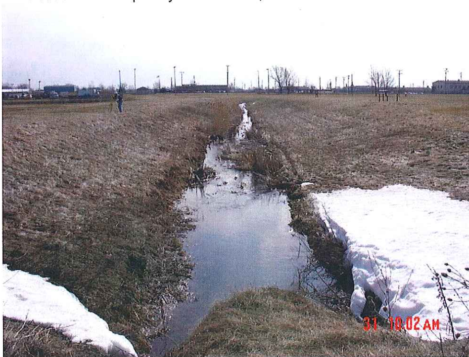
Stream downstream of bridge #2
