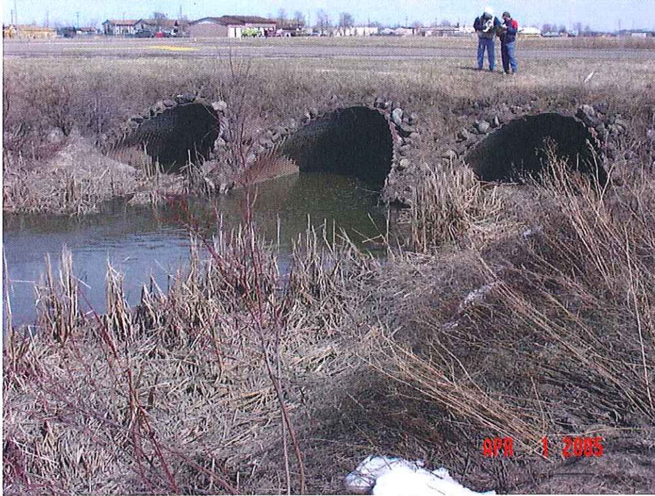
Downstream face of Bridge # 9
