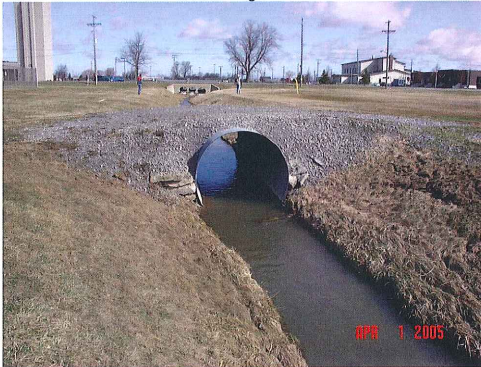
Downstream face of Bridge #5
