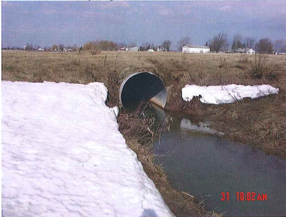
Downstream face of bridge #2 Photo Set #5 (Cross section #4)
