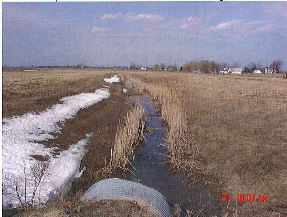
looking upstream from bridge #2 – cross section #3 is located upstream
