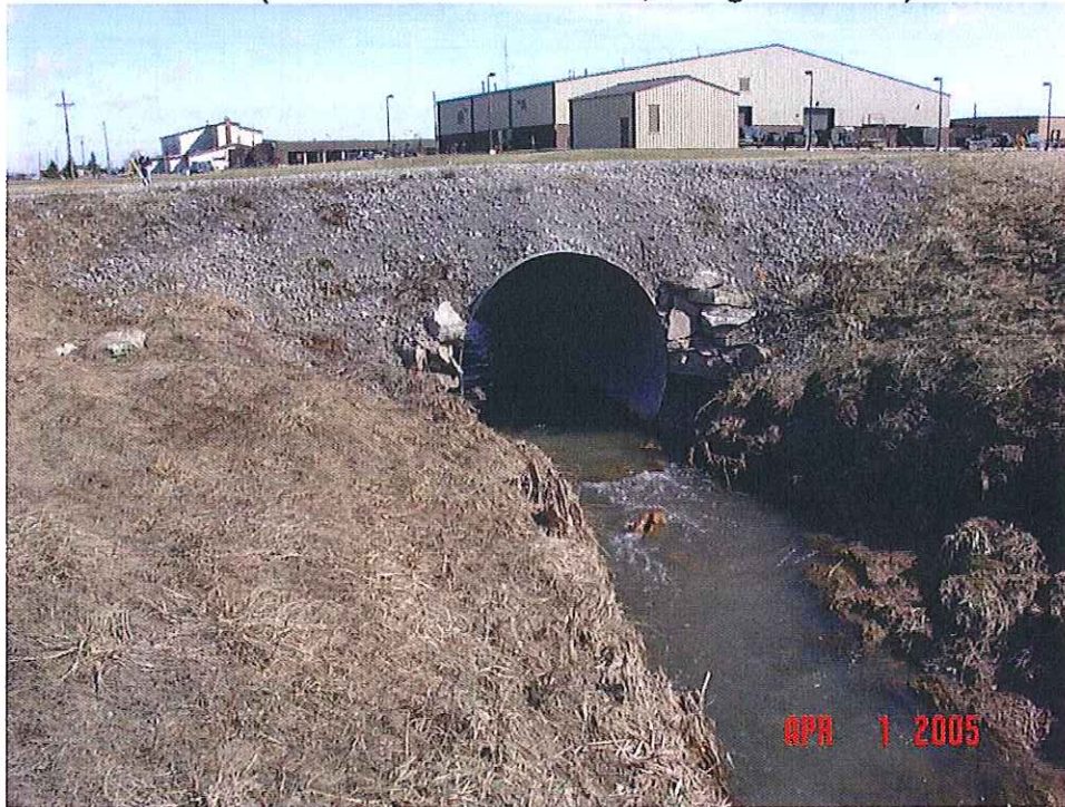
Downstream face of Bridge #6
