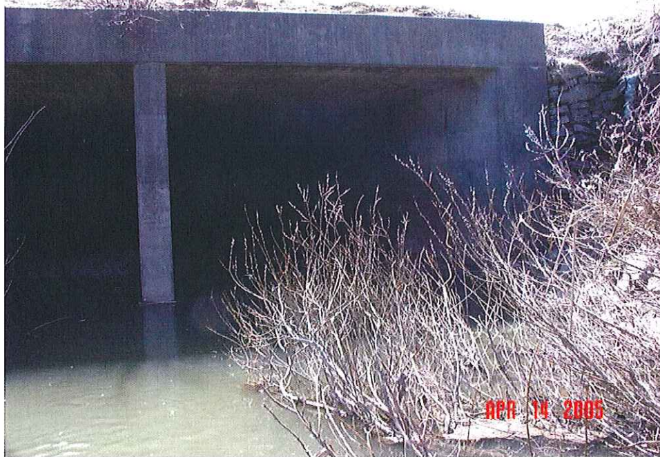
Upstream face of Bridge #10 – right half
