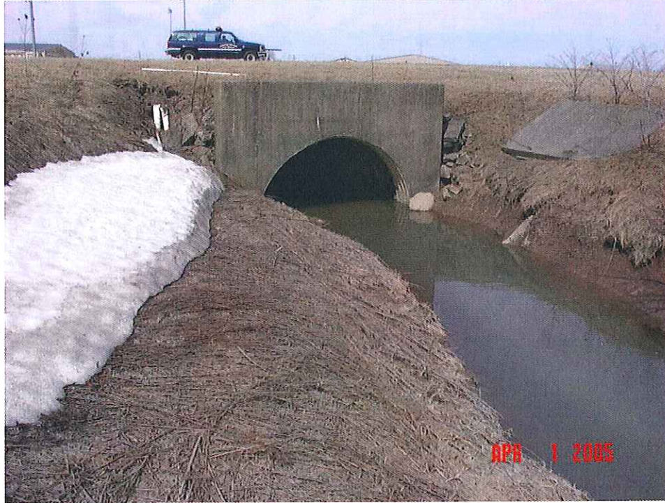
Downstream face of Bridge #8
