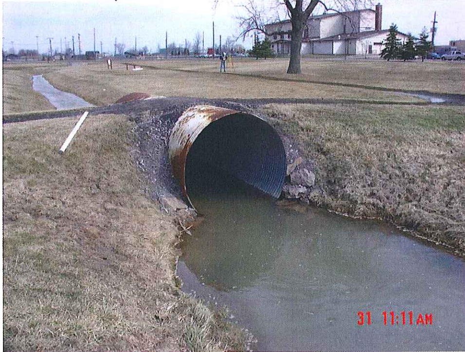
Downstream face of bridge #3
