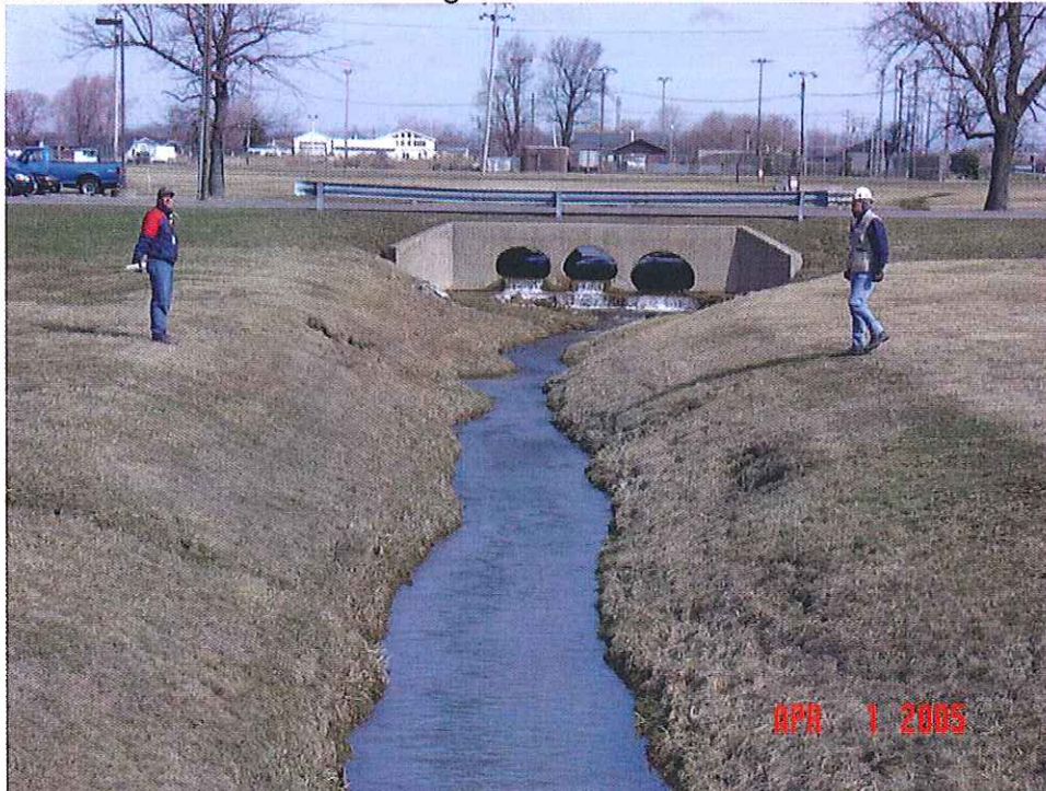
Looking upstream from Bridge #5
