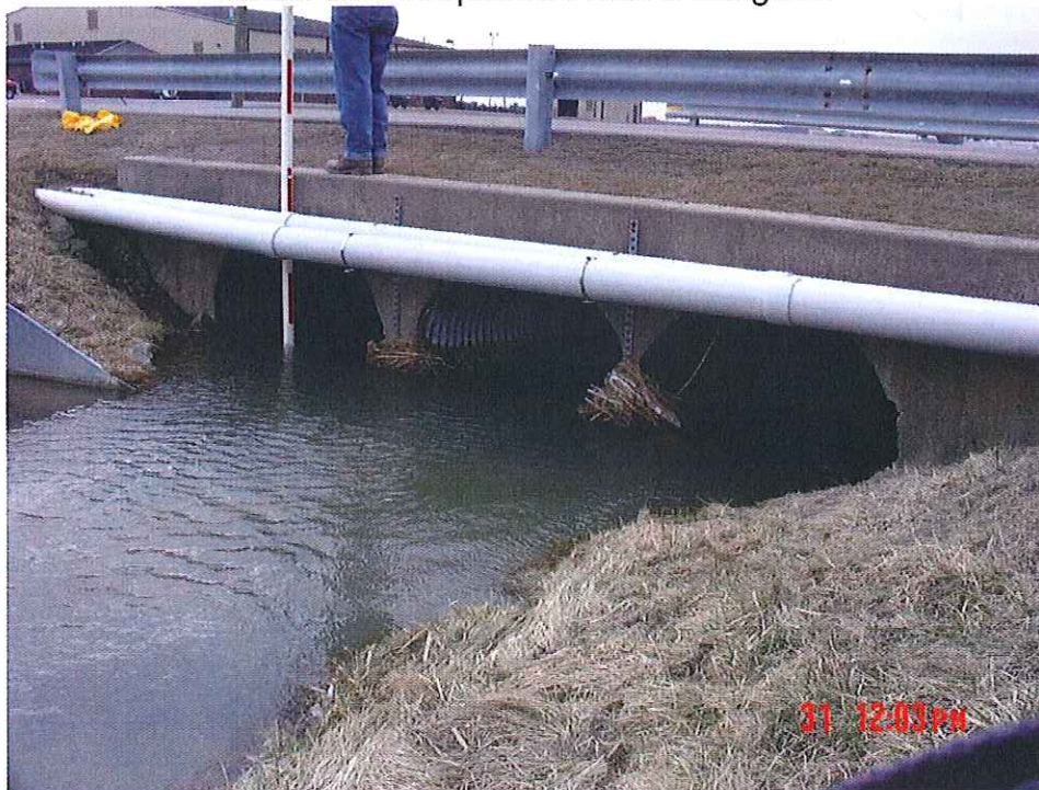
Closer view of upstream face of bridge #4
