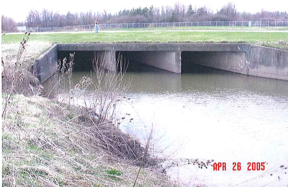
Upstream face of Bridge #11
