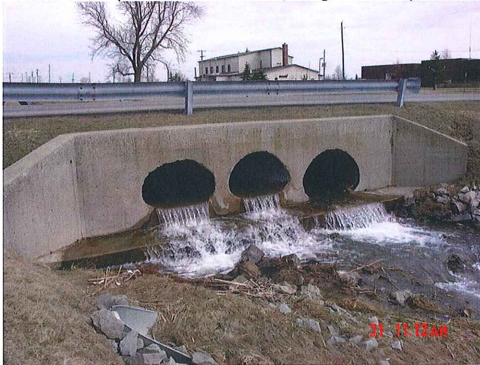
upstream face of bridge #4
