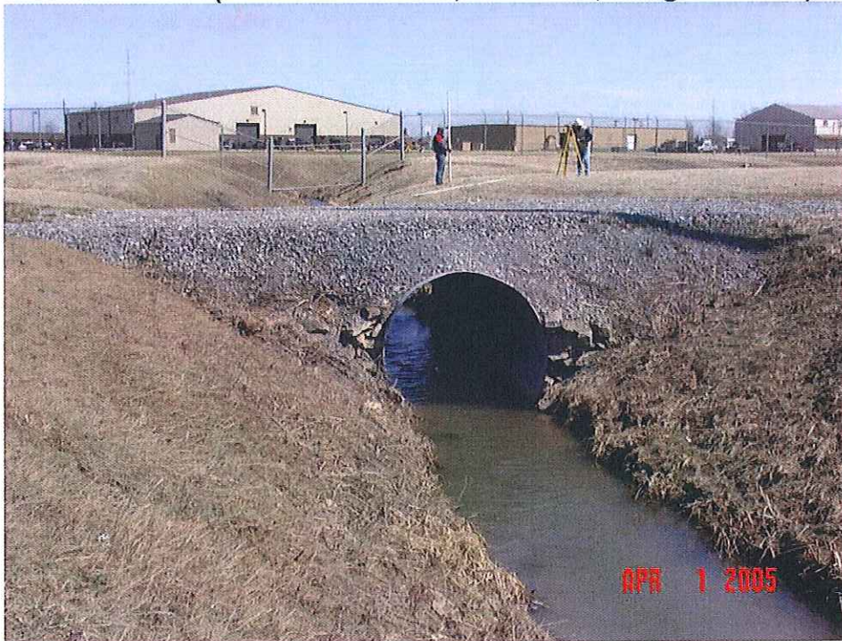
Downstream face of Bridge # 7
