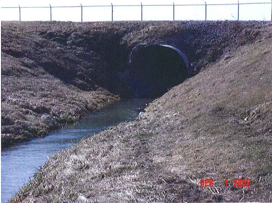
Upstream face of bridge #6
